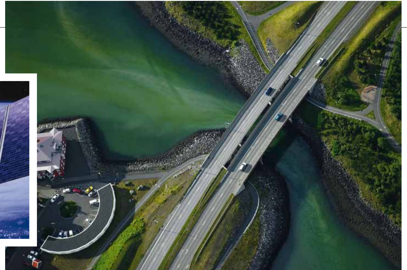
(Above, left) GALILEO, the GNSS built by the EU and the European Space Agency (Above right) GNSS facilitates accurate, flexible tolling operations
